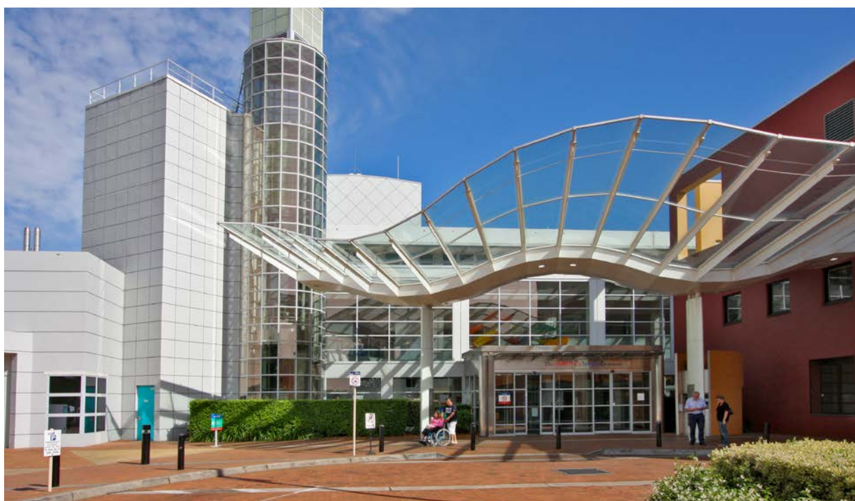
The Children's Hospital at Westmead
