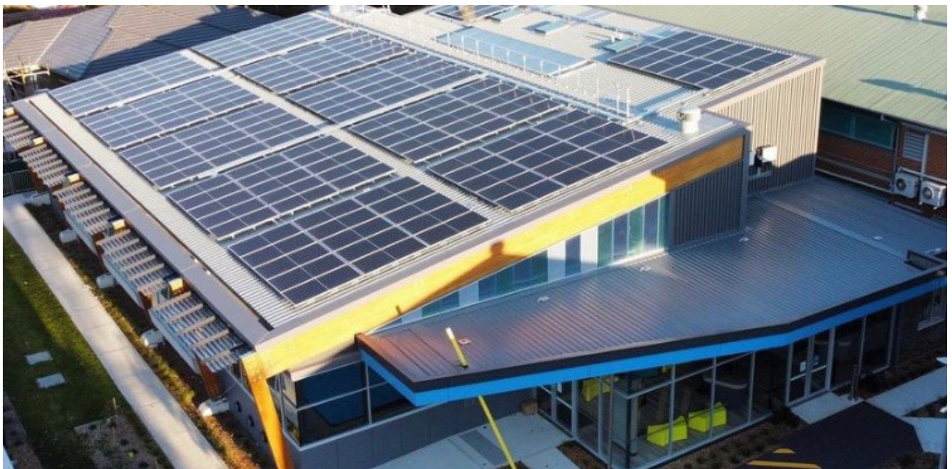
The Royal Life Saving Aquatic Safety Training Academy – Denistone East has 170 photovoltaic panels to convert sunlight to energy. In addition, there are 8 solar panels (pre-heat water) and 3 skylights to add natural light to the mezzanine level. The facility was officially opened in June 2021.
